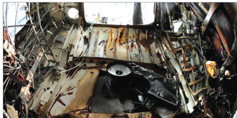
〈Figure II-2-10〉 Bulkhead between gas turbine room and diesel engine room
